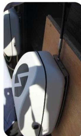
Replace the locking plate and screws to secure the unit. Power up the unit and test.
