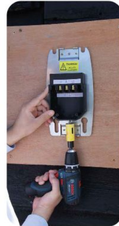
Using a hole cutter, cut a hole into the benector the correct size for the gland.
