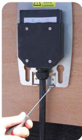
An additional screw is provided should you need another earth connection.
