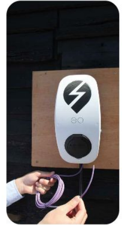
Offer up the charger to the base plate. (If installing an eoGenius ensure that the data cable does not get trapped).
