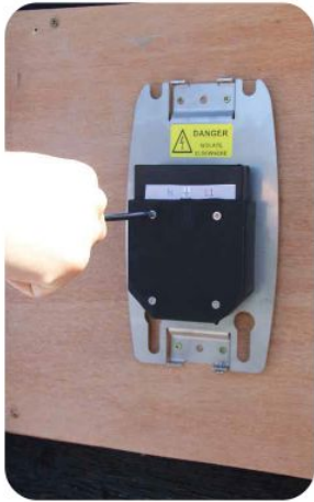
Unscrew the cover on the benector.
