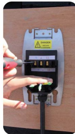
Unscrew the 6 screws (10 screws if installing a 3-phase unit), feed the cable through the gland and secure. Prepare the ends with ferrules.
